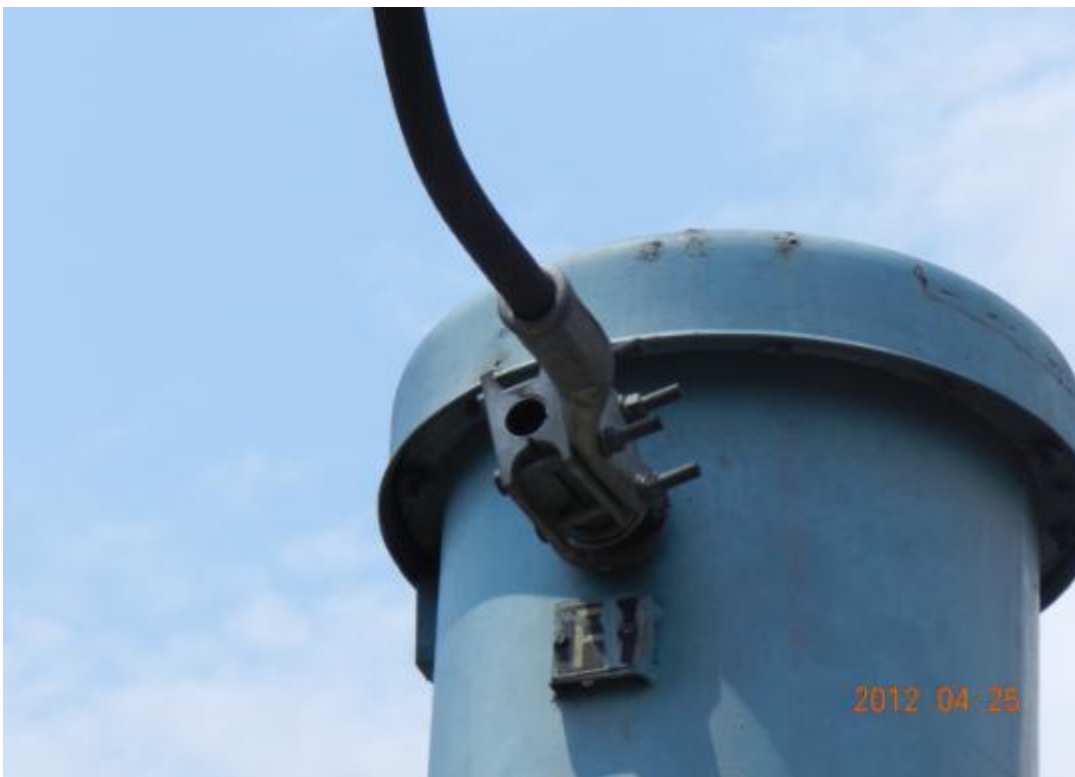
11.CT CONNECTOR FOR MOOSE CONDUCTOR
