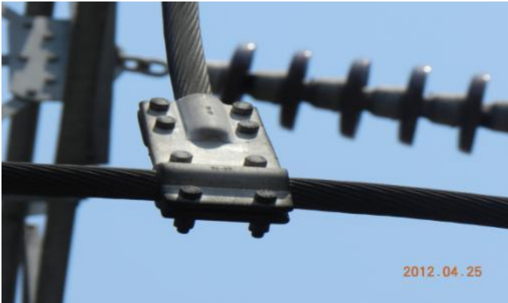
11.CT CONNECTOR FOR MOOSE CONDUCTOR
