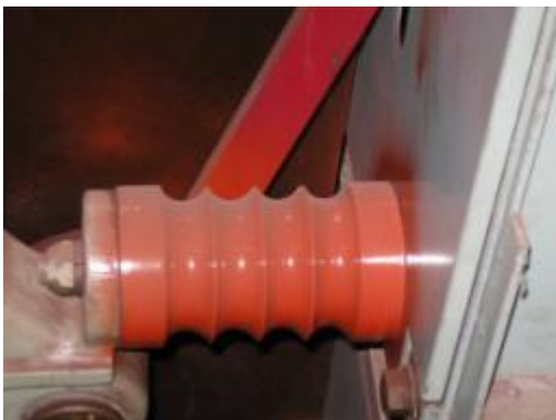
EPOXY INSULATOR FOR 6.6KV VCB
