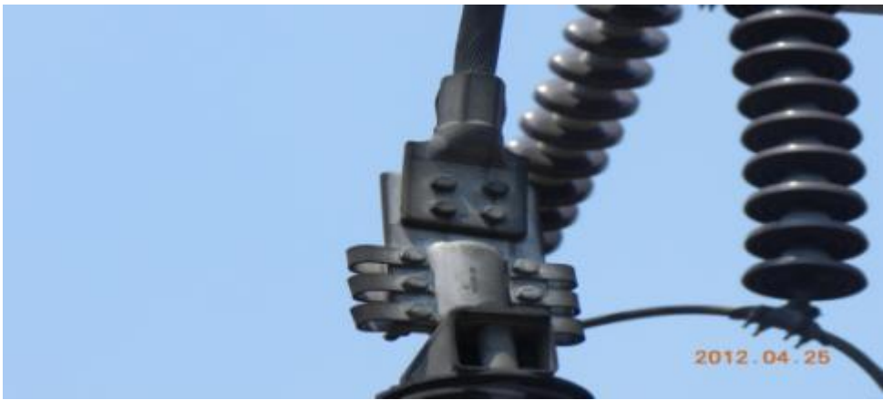
4.BREAKER CONNECTOR FOR MOOSE CONDUCTOR
